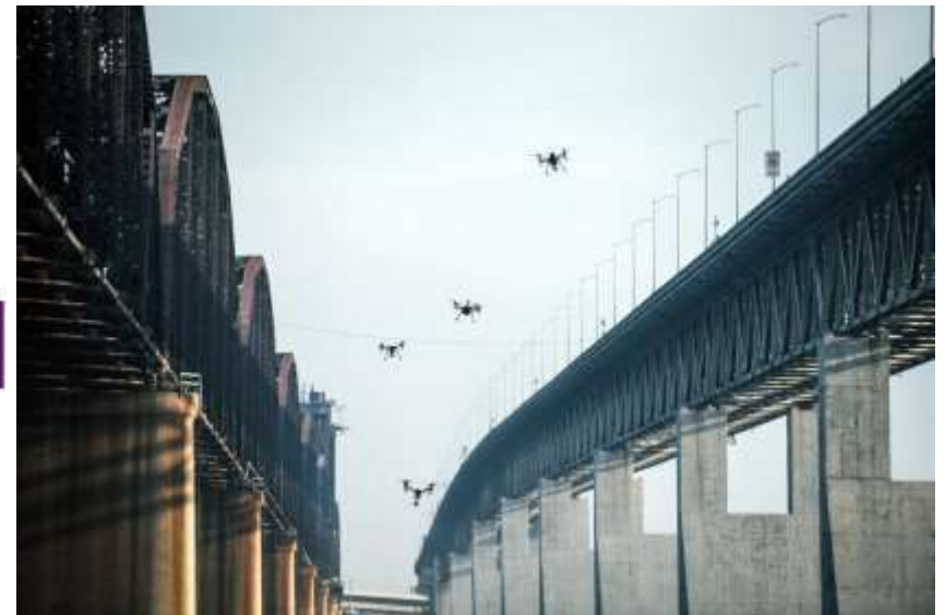
Autonomous drones are tested as the railroad bridge adjacent to the Benicia-Martinez Bridge in California.
